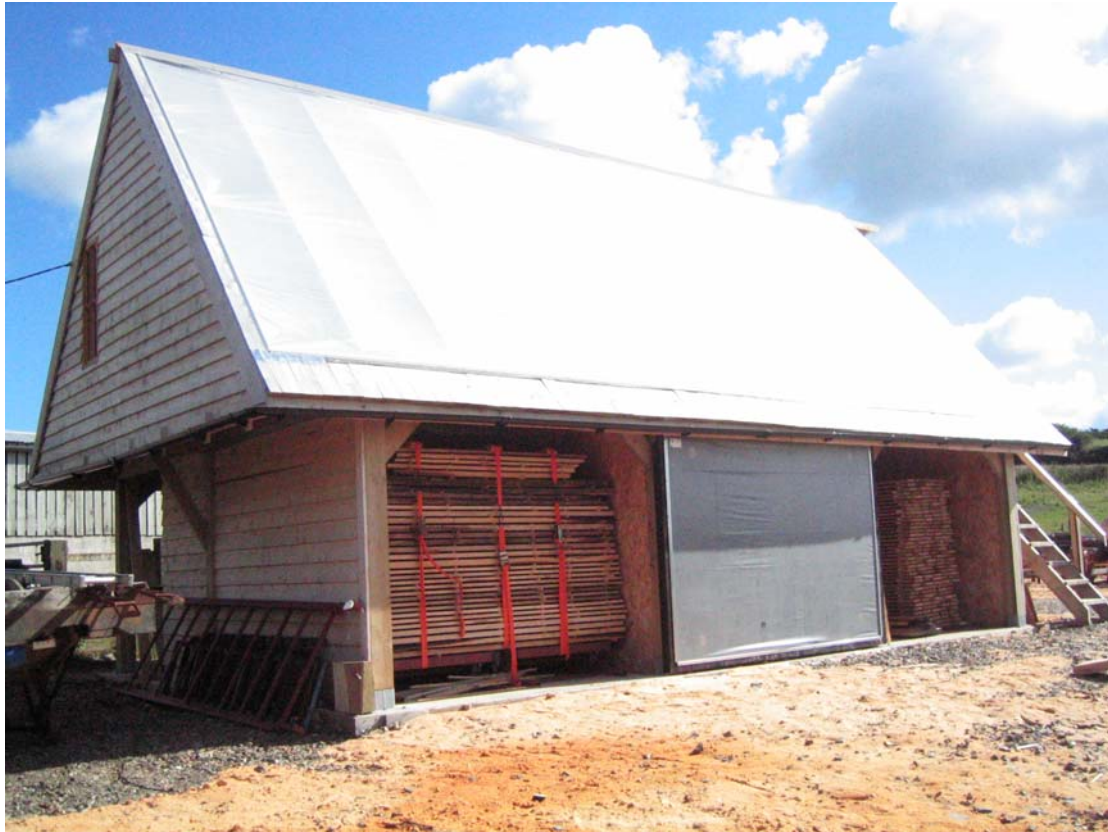
The Solar Wood Drying Kiln
